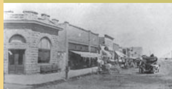
This preserved historic Driggs building reinforces a strong sense of place and community character.
