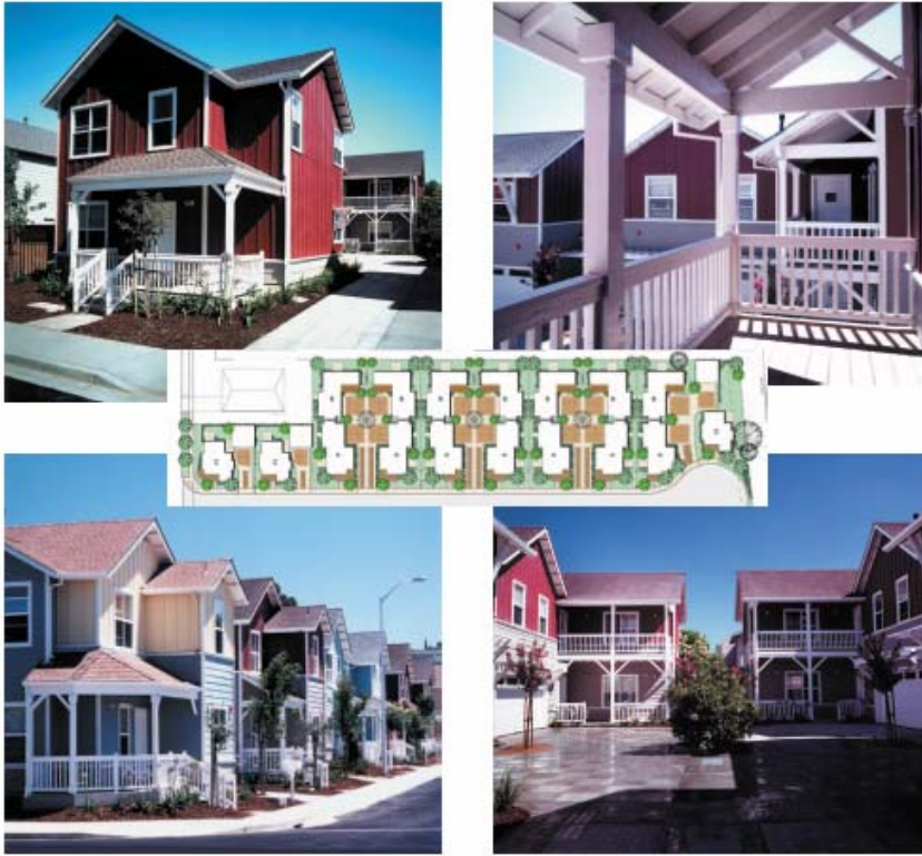
Figure 30: Single family homes built on small lots in the Irvington neighborhood of Fremont, California
