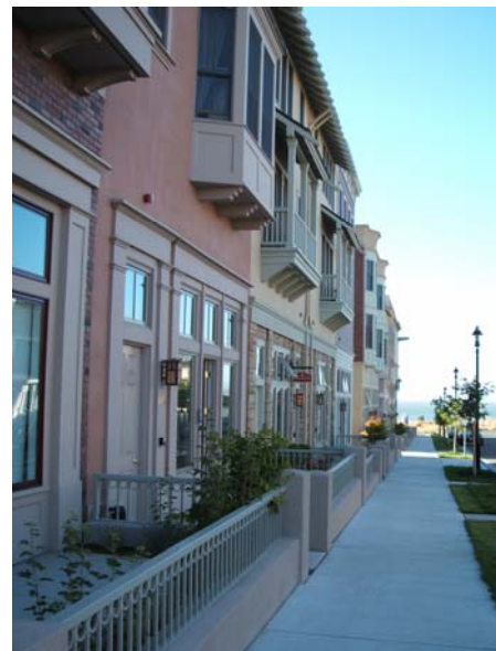
Figure 33: Live-work homes, Hercules, California
