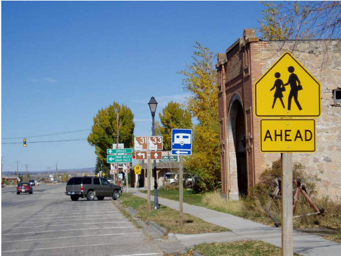
Figure 15: Main Street in Victor looking north showing the basic design elements of a good pedestrian realm – roadway corridor with diagonal parking, planting strip, sidewalk, and setback
