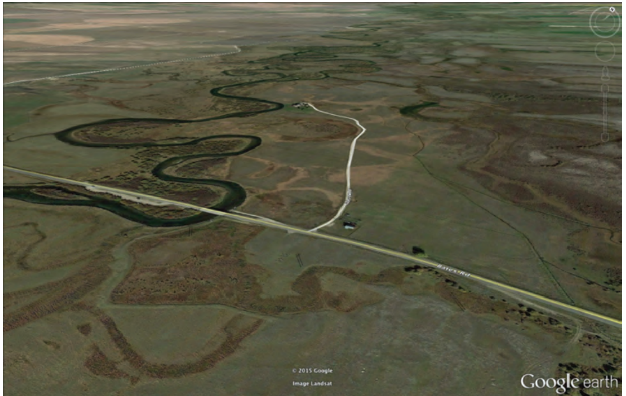
Area near Bates Road at Bates Bridge
