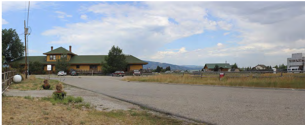
Existing Conditions. Looking west down Depot Way towards the train depot.
